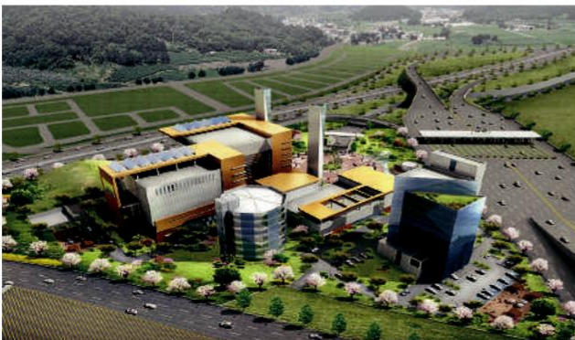
Cogeneration Plant 210RT 4units, 180RT 3units
