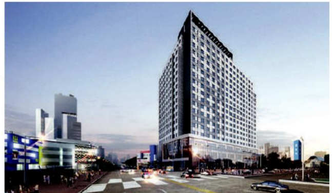
Harrington Tower 240RT 5units
