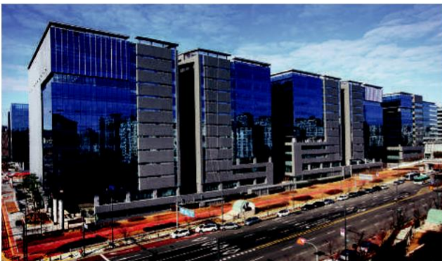
Korea Venture Town 340RT 6units, 300RT 4units
