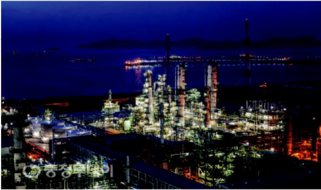
Lotte Chemical Industry 1300RT 3units, 975RT 1unit
