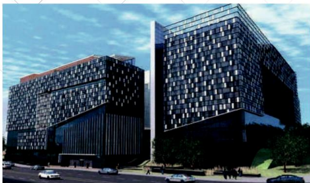
Pangyo CHA Hospital| Institute 675RT 3units
