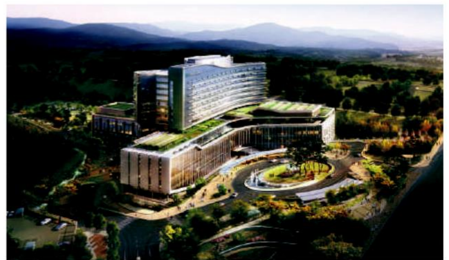
GyeongSang Univ. Hospital 300RT 2units
