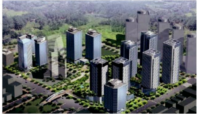
International Building 500RT 2 units, 560RT 2units, 150RT 2units
