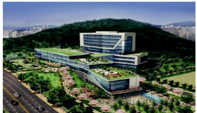
Daegu Regional Government Complex 420RT 2units
