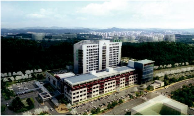
Ilsan Hospital 900RT 2units, 300RT 1unit
