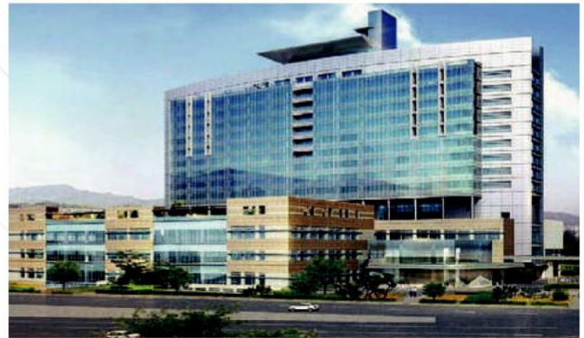
Hanjin University Hospital 900RT 2units
