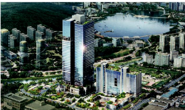
IT Valley 825RT 5units, 270RT 3units
